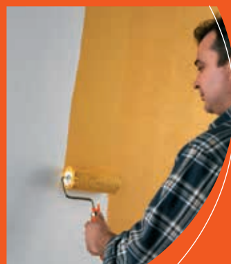
3 - After the glue has completely dried, apply two layers of quality paint
