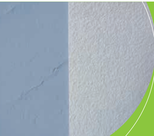
RenoLisse applied over medium size crack
