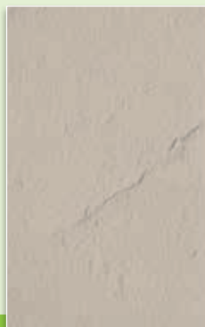
Medium cracks
